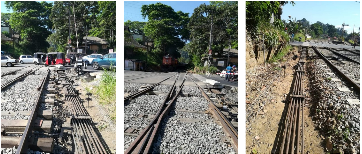
PDA Level Crossing Rehabilitation
