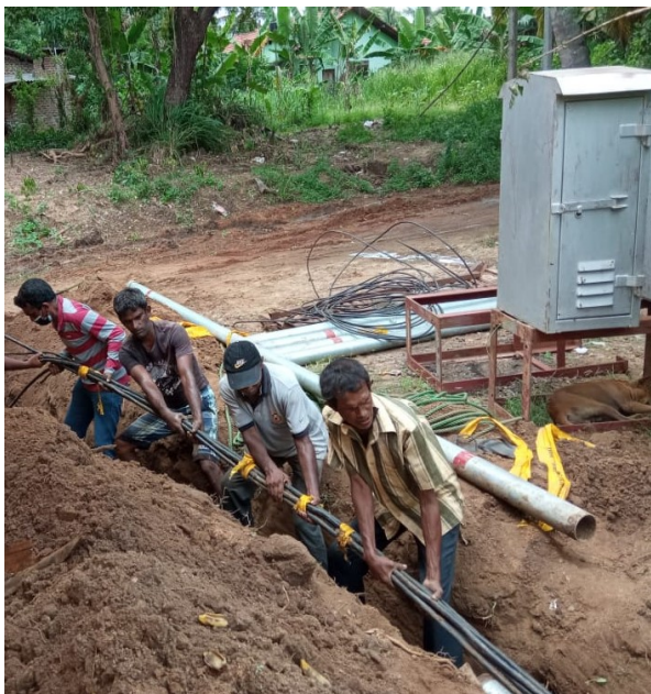
Cable Laying Works at WEL
